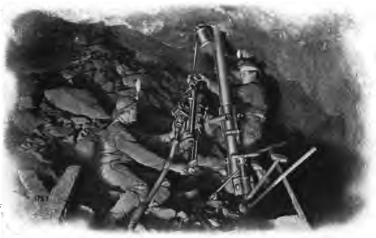
BALTIC MINE.—FILLING SYSTEM. Showing Method of Stoping on Top of Filled Ground.
